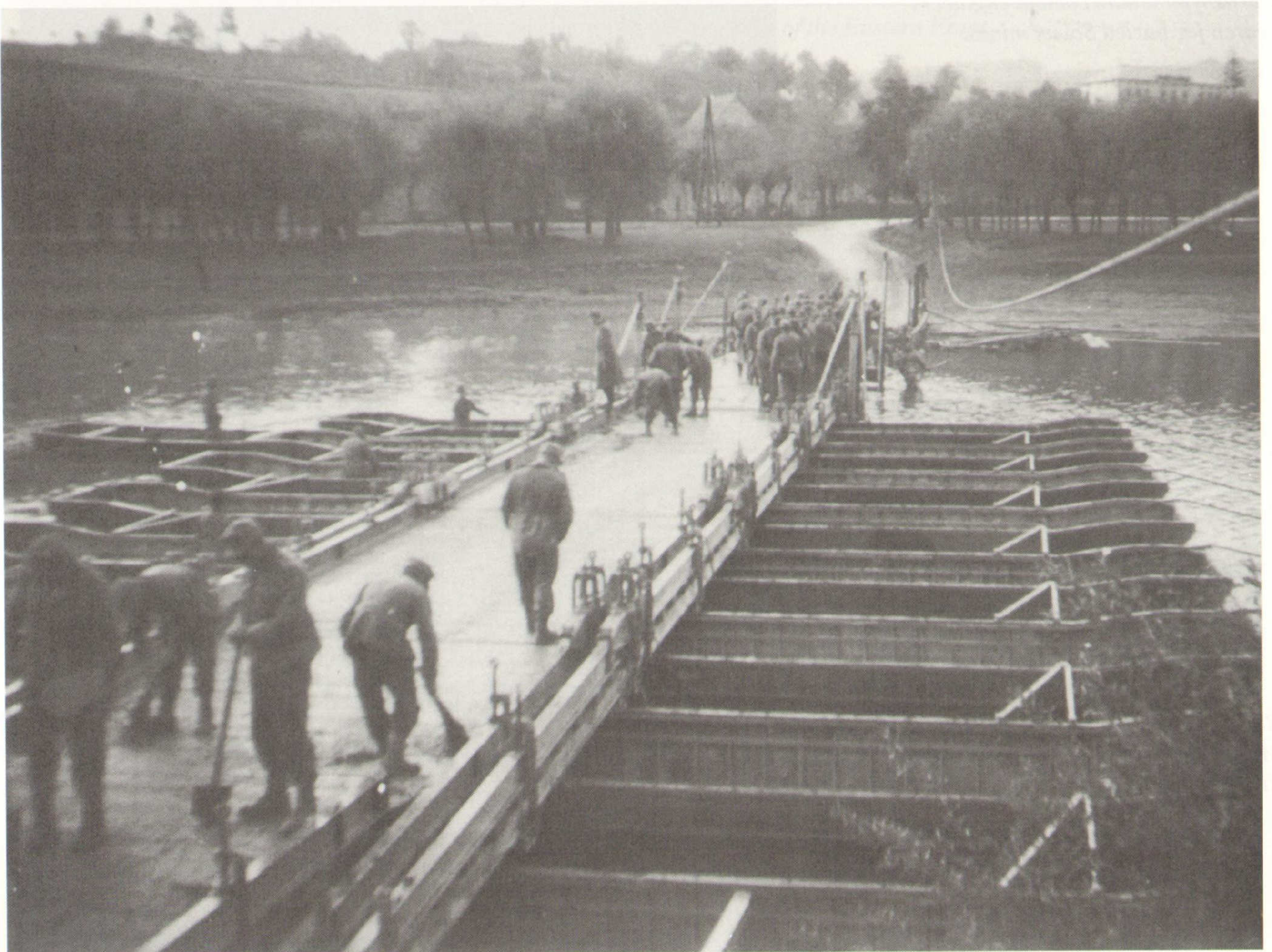
Construction of a military bridge by Gebirgstruppe combat engineers in France in 1940.
